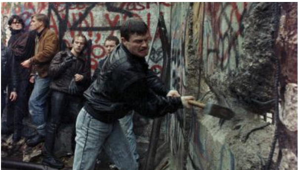
Demolition of Berlin wall
